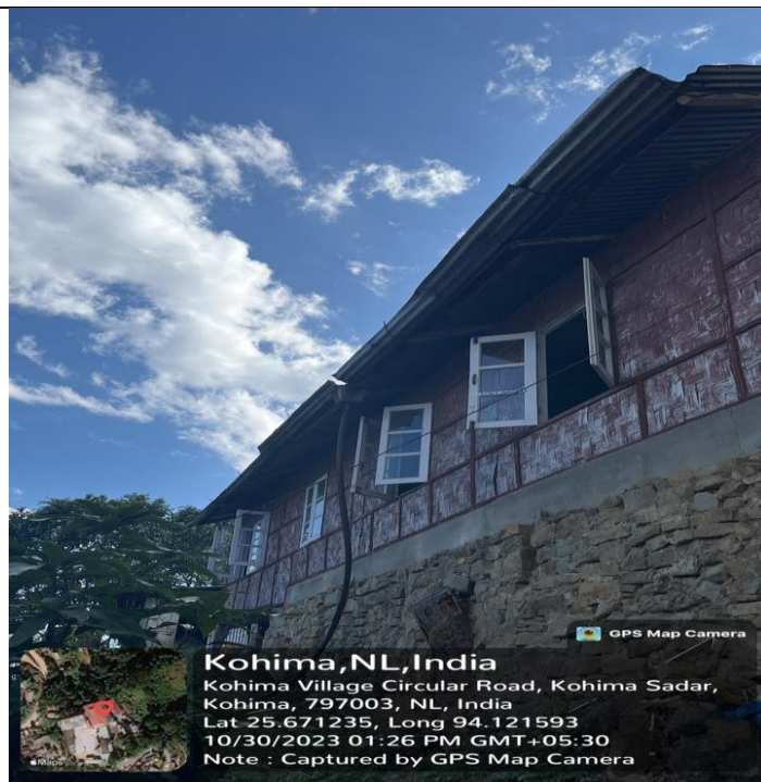
Rainwater harvesting in lower block classrooms
